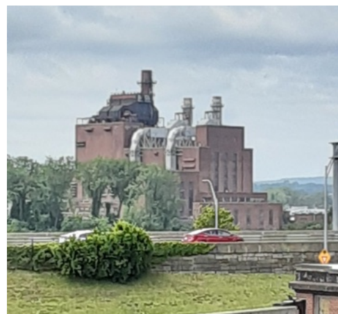
West Springfield peaker plant, soon to be transitioned to renewables
