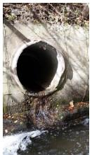
the rate of flow as "moderate", the odor as "sewage", and the condition as "minor damage". What's more, there is a sewer line running past the outfall. Also, this outfall did not appear on the City of Pittsfield's Storm Water System map or GIS layer. Due to these characteristics, BEAT decided to sample this outfall.
